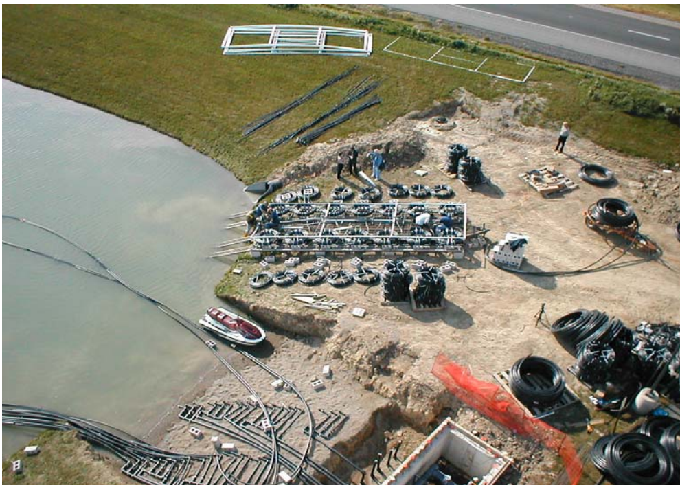
Fig. 1. Pond loop for system integration. Loop is high density polyethylene (HDPE), rated capacity is 150 kW, pipe bundles are fabricated from 19-mm pipe with spacers between loops. Each bundle has 92 meters of pipe. Header pipe sizes to and from building are 0.19 meters. Photograph courtesy of Geothermal Design Associates Inc. Ft. Wayne Indiana
