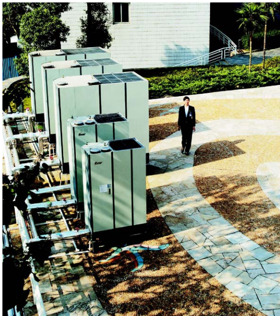
Fig. 3. Five BCT Units ranging from 16 kW (foreground) to 115 kW center)
