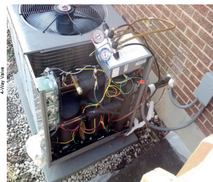
Annex 41: 2015 CCHP field test; single-stage vapor compression cycle with dual single-speed compressors – schematic (left image) and field test prototype system installed in late January at residence in Ohio. [Source: Oak Ridge National Laboratory and Copeland Compressor]
