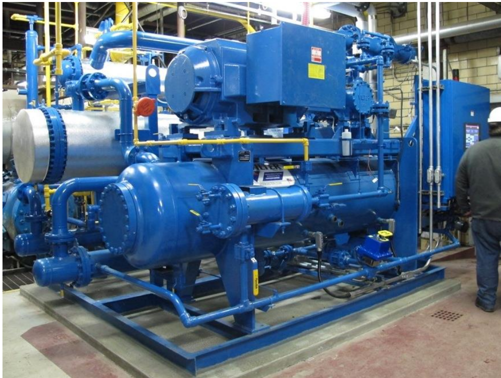
Figure 9. Single Screw Heat Pump System for Food Plant Sanitation
