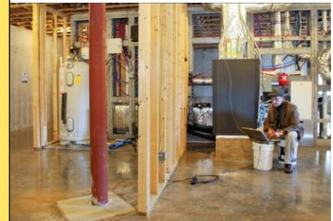
Prototype GS-IHP installed in test house
