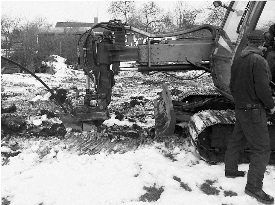
Figure 4. Machine for ploughing and tube placing in one operation
