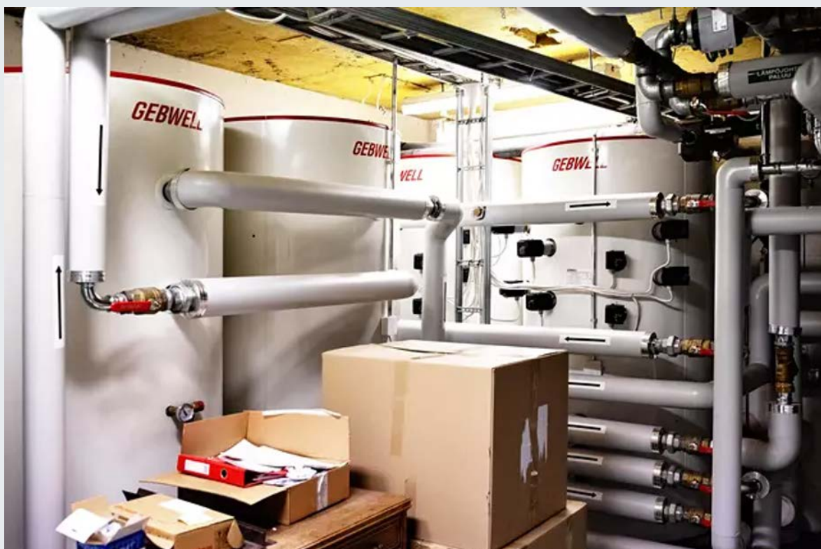
Fig. 3: Geothermal heat is local heat, originating from the rock on which the houses are built. With these devices, heat is pumped from the earth's crust. Photo: K. Rautaheimo, Helsingin Sanomat.
