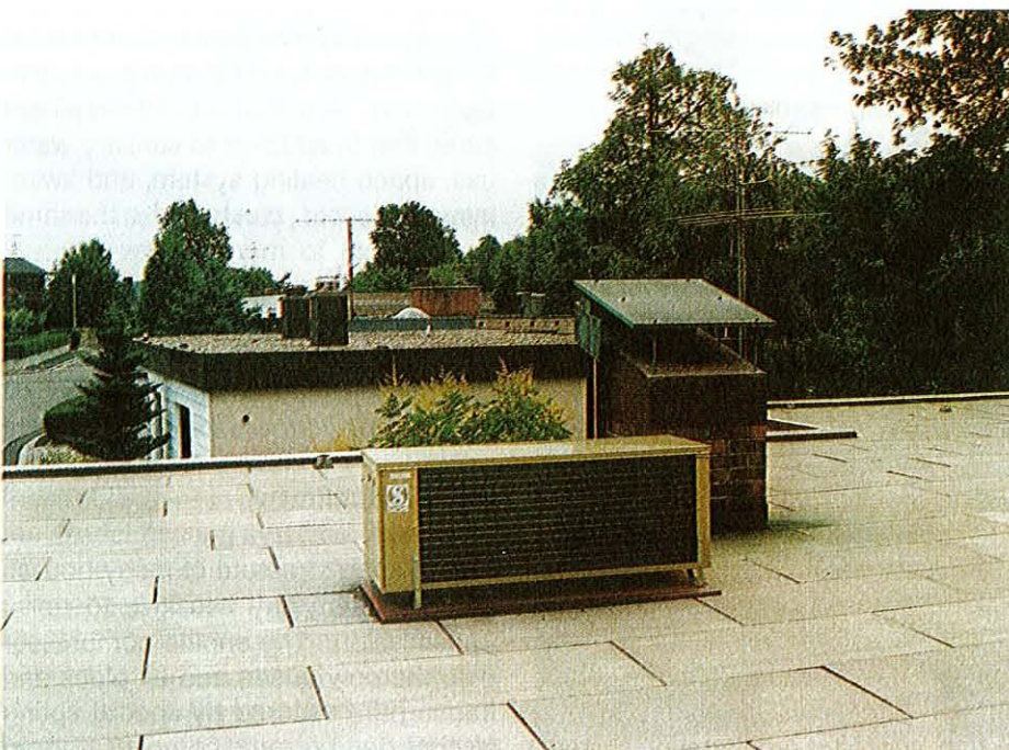
Figure 3. Roof-mounted Sachs air evaporator
