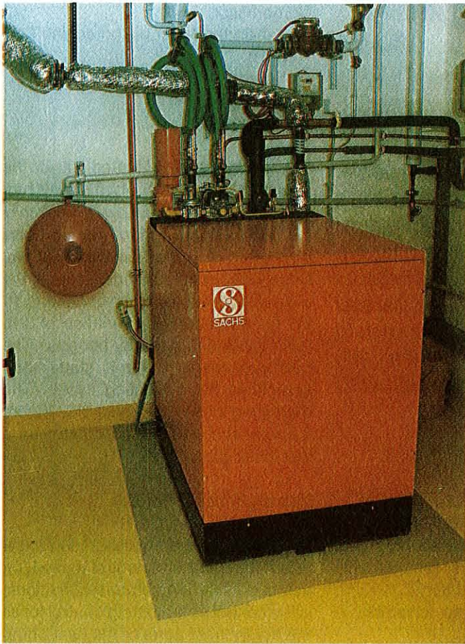
Figure 1. Sachs heat pump installed in a residence with a 50kW heat load
