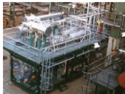
▼ Figure 3: Absorption refrigeration unit equipment skid.
