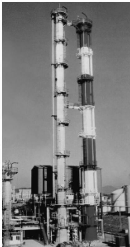
▲ Figure 1: A distillation plant with heat pump in Ulsan, South Korea, that separates 1-butene.
