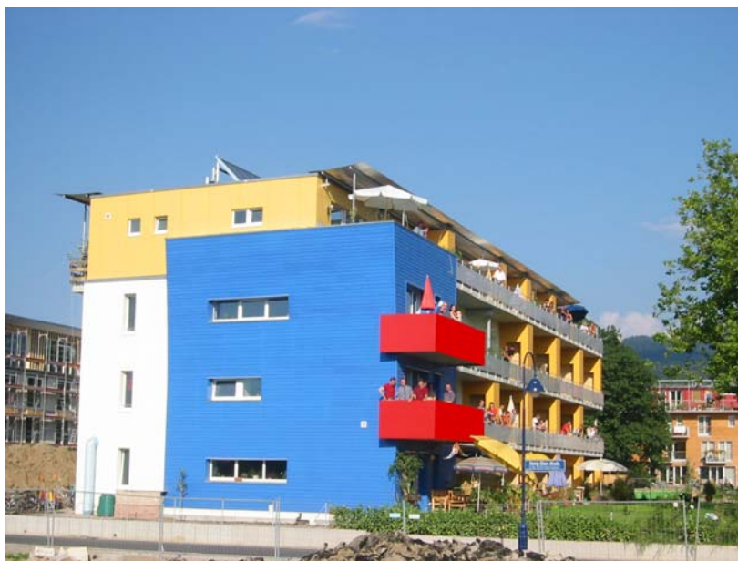
Fig. 1. Example of a Solar Passive House. This multiple family dwelling has been erected in the new Freiburg area Vauban. The heating demand meets 10 \text{ kWh}/(\text{m}^2\text{a}) . The apartment in the foreground (author's flat) is supplied by a newly developed compact heating and ventilation device with integrated exhaust air heat pump.
