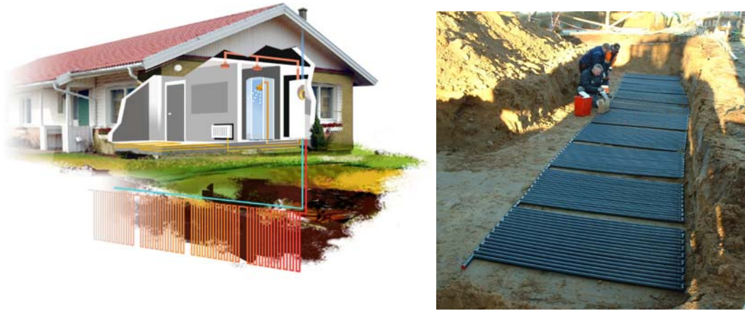
Fig. 8. Vertical and horizontal installation
