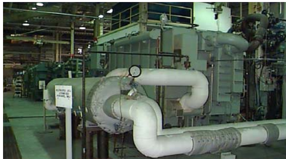
Fig. 4. Triple effect, indirect-fired absorption chiller tested at York International, York, Pennsylvania.
