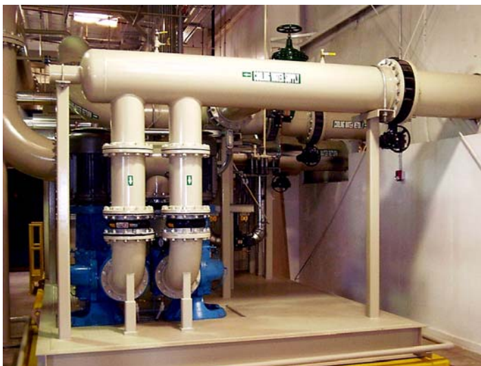
Fig. 1. Burns & McDonnell IES in Austin, Texas With a Direct Exhaust Fired Absorption Chiller
