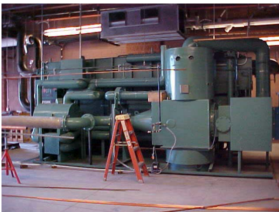
Fig. 5. Triple effect, direct fired absorption chiller installed at the Clark County Government Center, Clark County, Nevada.
