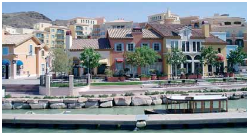
Lake Las Vegas with water-source heat pumps.
