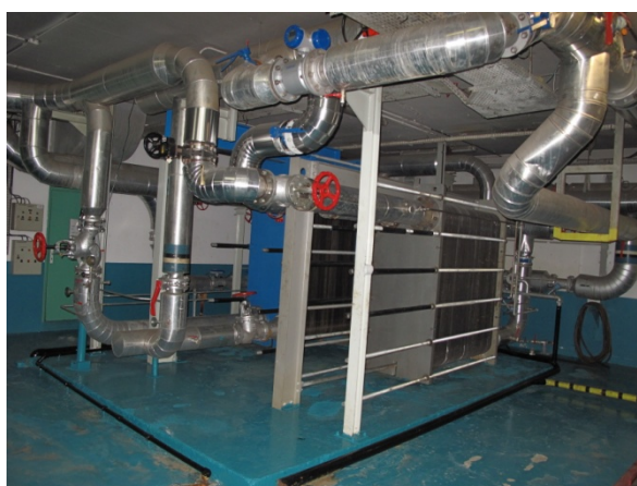
Figure 9: Titanium heat exchangers of a geothermal installation with Dogger water.
