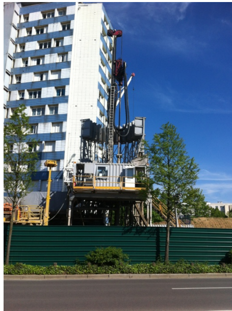
Figure 7: Borehole drilling of injection well (Le Plessis-Robinson).
