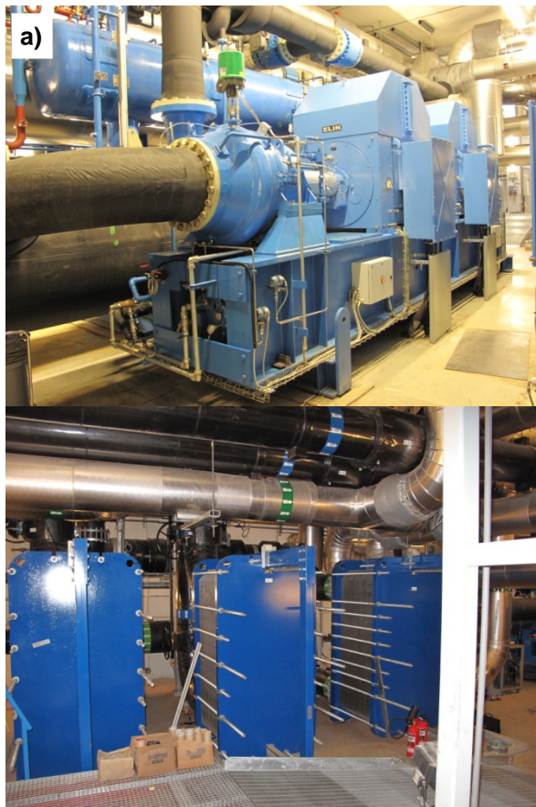
Figure 4: a) UNITOP 43/28 installed in the Rolfsbukta heat pump plant, b) Intermediate heat exchangers between sea and clean water.
