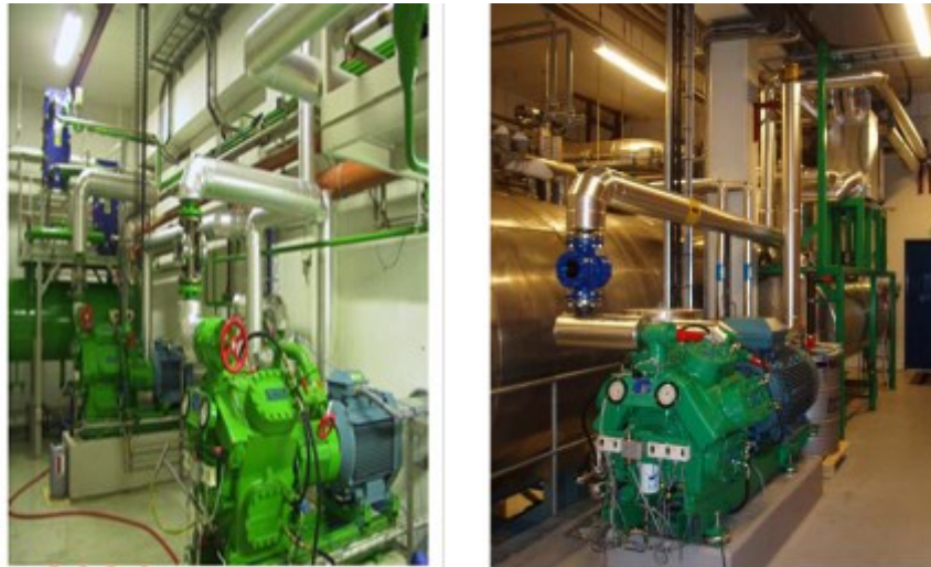
Figure 2: Pictures of two “hybrid” heat pumps by “Hybrid Energy AS” left: 300 kW, right: 650 kW heating capacity (Nordtvedt 2009)
