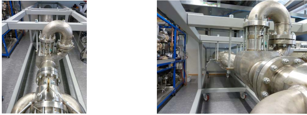
Fig. 8 Thermo acoustic heat transformer at ECN
