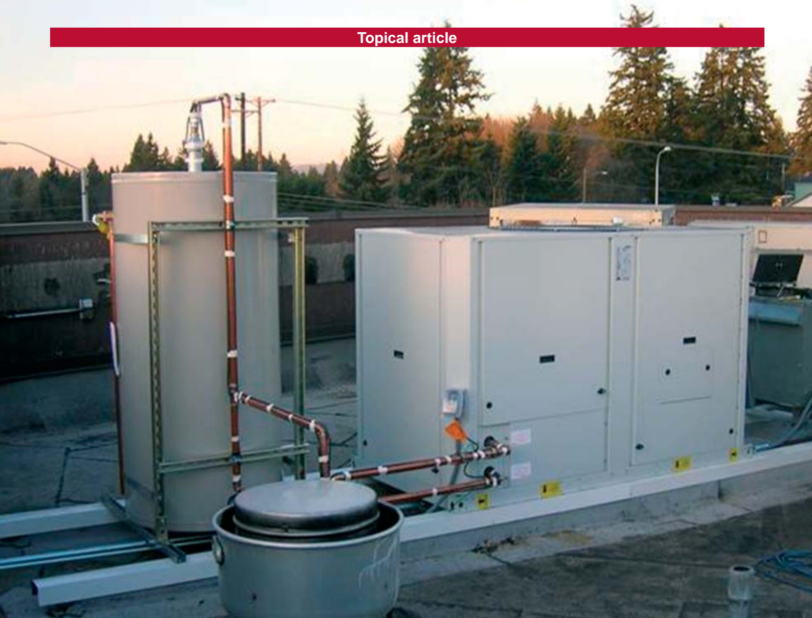
Figure 3 – Carrier 60kW CO 2 Heat Pump installed on restaurant roof in Oregon
