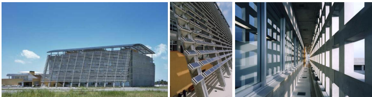
Fig. 18: The building's exterior view (left), Amahaji style eaves (middle) and perforated PC paneling on western face (right)
