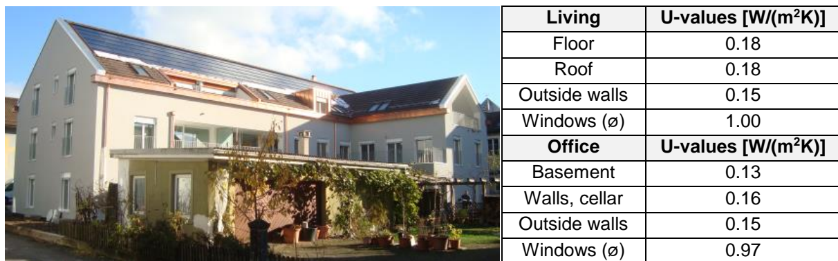
Fig. 59: Monitored MINERGIE-A® building in Uster and envelope characteristics (Hässig, 2013)
