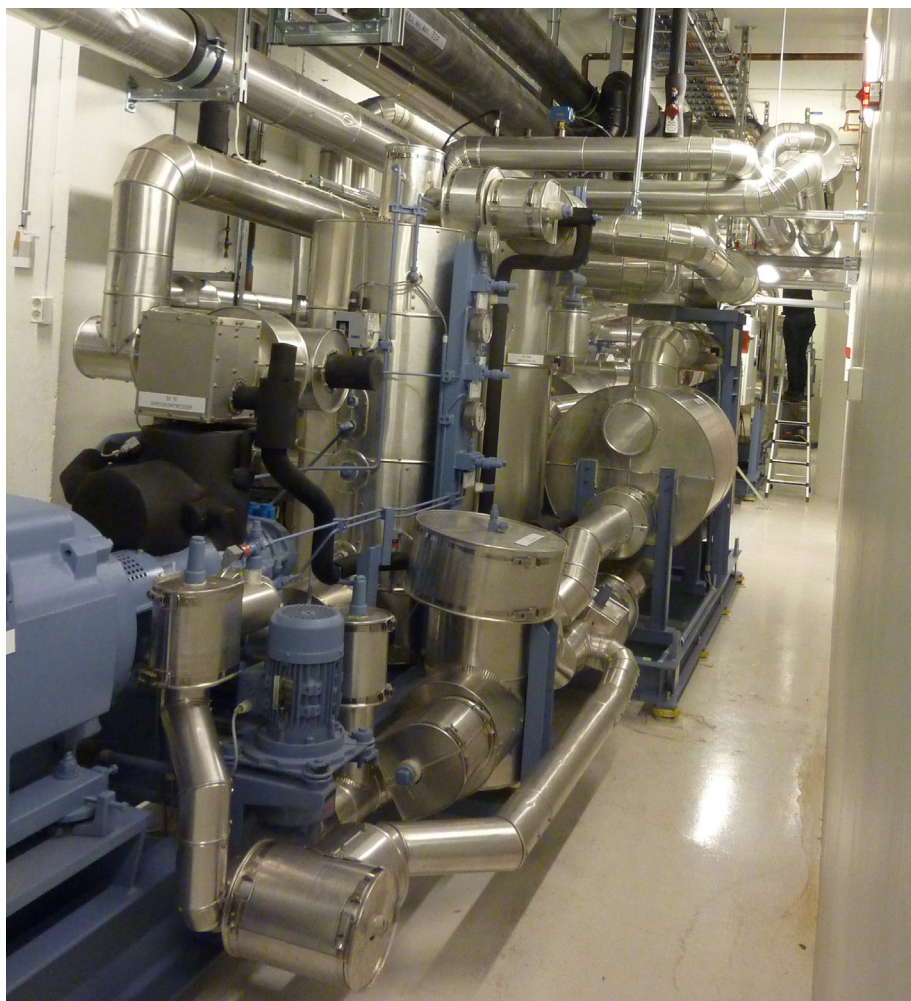
Figure 3. High-temperature liquid chiller and heat pump unit with variable speed drive twin-row compressor [Photo: Eptec Energi AS]
