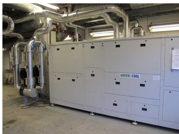
Figure 2. 350 kW CO 2 HPWH at UNN. Photo – Kuldeteknisk AS.
