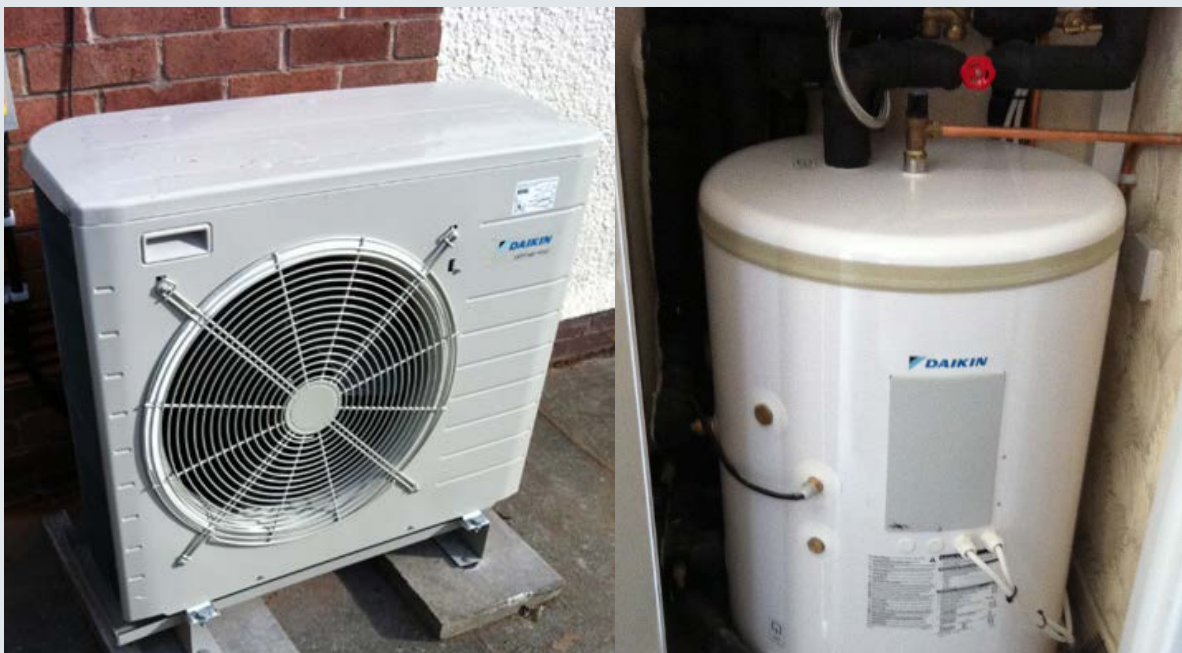
Figure 4. Heat Pump Unit introduced in Public Houses in Manchester (UK)
