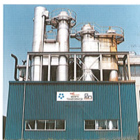
Figure 9 (bottom left): This Absorption heat pump supplies a district heating system using energy from high and low-temperature heat streams from a chemical process.
