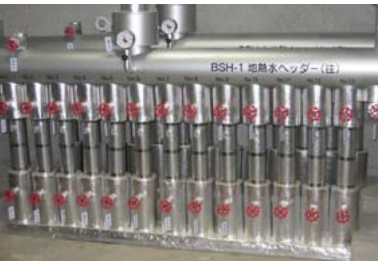
GSHP supply header in Sapporo City University.
