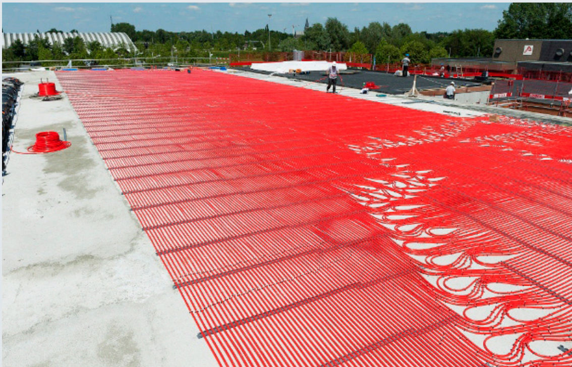
Figure 2. Build-up of the energy roof.
