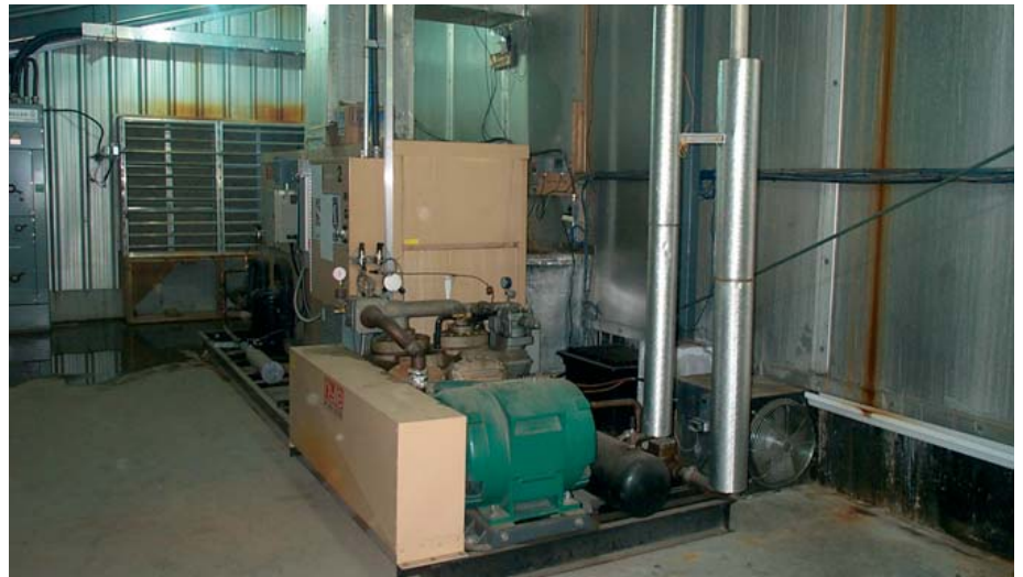
Photograph 1 – View of one of high-temperature heat pump prototypes
