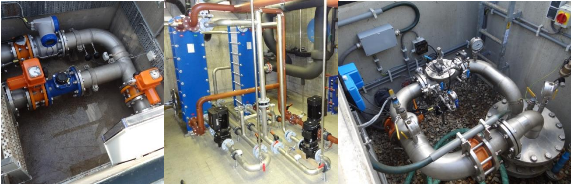
Fig. 8. left to right: DATES Connection point, building delivery set, “old” well with new reinjection valve
