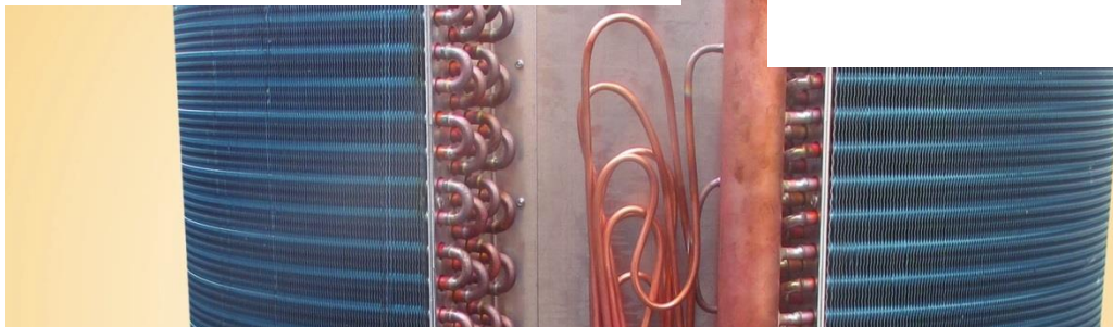
Fig. 1. Outdoor coils for residential heat pump are migrating towards smaller diameter copper tubes, to increase efficiency and reduce refrigerant volume. This MicroGroove coil uses 7-mm outer diameter copper tubes. (Photograph courtesy of Lordan.)
