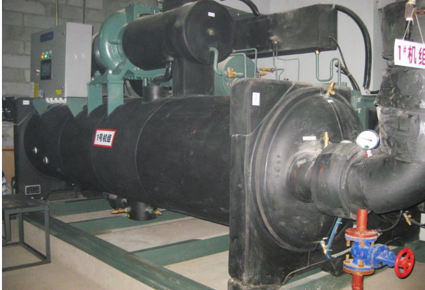
Fig.5 Field test site of district heating using PSF centrifugal heat pumps
