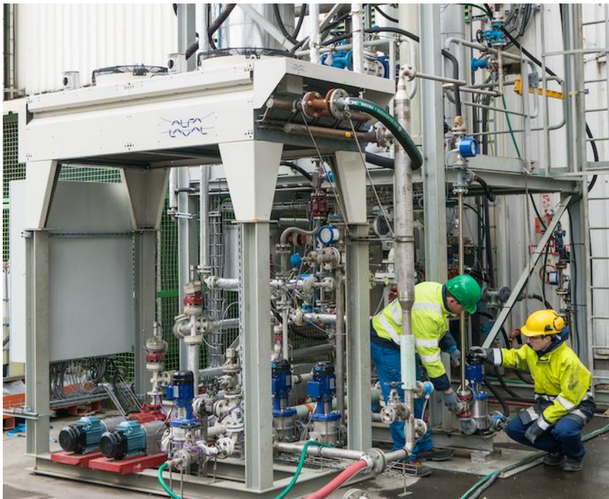
Figure 4 Working @ Qinch 50 kW output heat trafo at Indaver Antwerp, Belgium 2016
