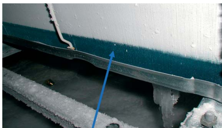
No frost formation or growth of freeze in the non-frost area
