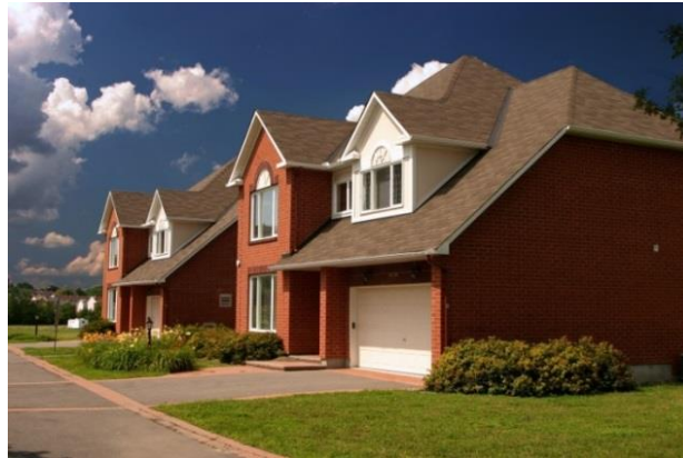
Fig. 2. Images of CCHT Twin House Test Facility
