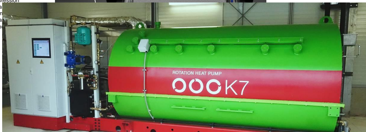
Fig.: 9 Implemented RHP K7 Pilot at Biomass Heating Plant©
