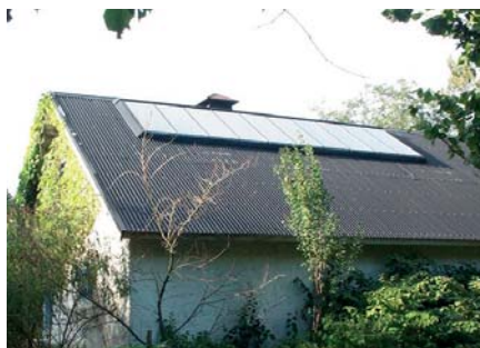
Fig. 2. Typical size of solar collectors on a single-family dwelling in Sweden in a combisystem for domestic hot water and space heating of the building.
