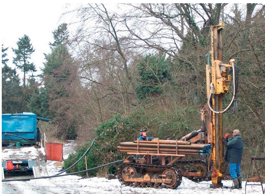
Figure 1. Drilling a borehole for a single family dwelling
