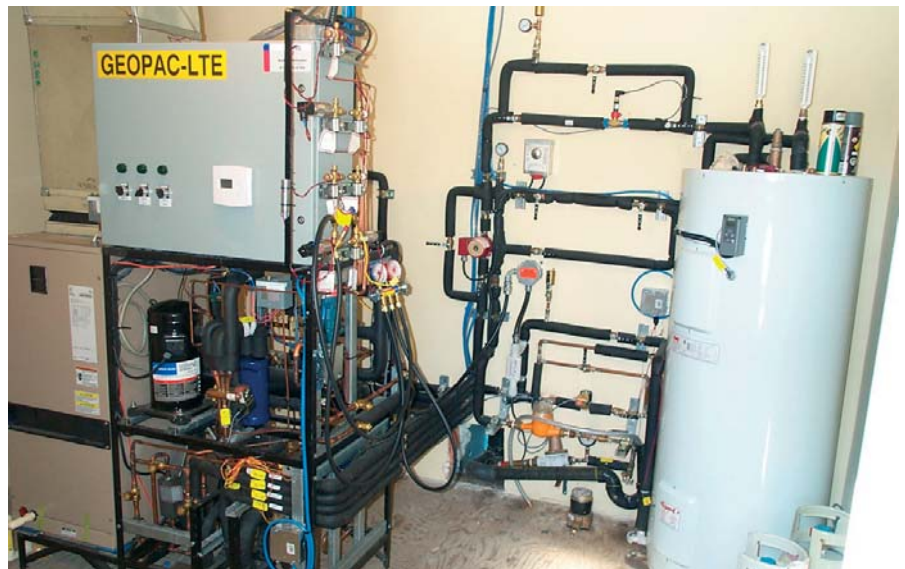
Photograph 1 – View of the combined multifunctional GSHP prototype (GEOPAC-LTE)
