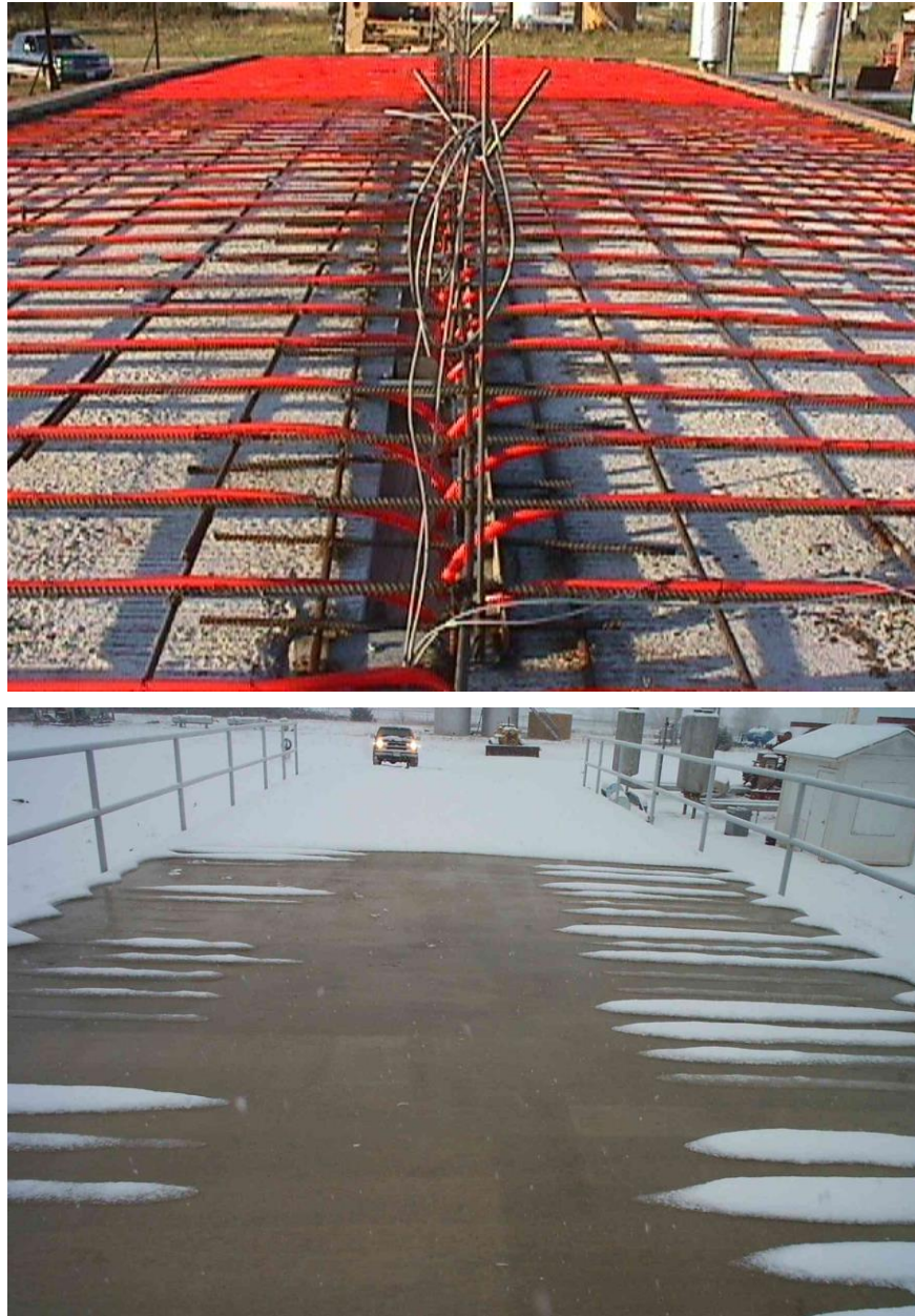
Figure 2 Geothermally Heated Bridge Deck at Oklahoma State University. Above: Before concrete has been poured with hydronic tubing visible. Below: Near the end of a 200 mm snow fall in December of 2000, with heated portion in foreground
