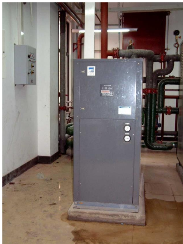
Fig. 7 Ebara screw heat pump on the site
