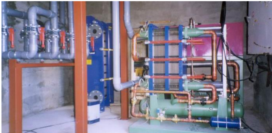
Photo 2. High efficient heat pump system of supply seawater volume 40 m 3 /h using seawater and exhaust water heat source in land based aquaculture system.
