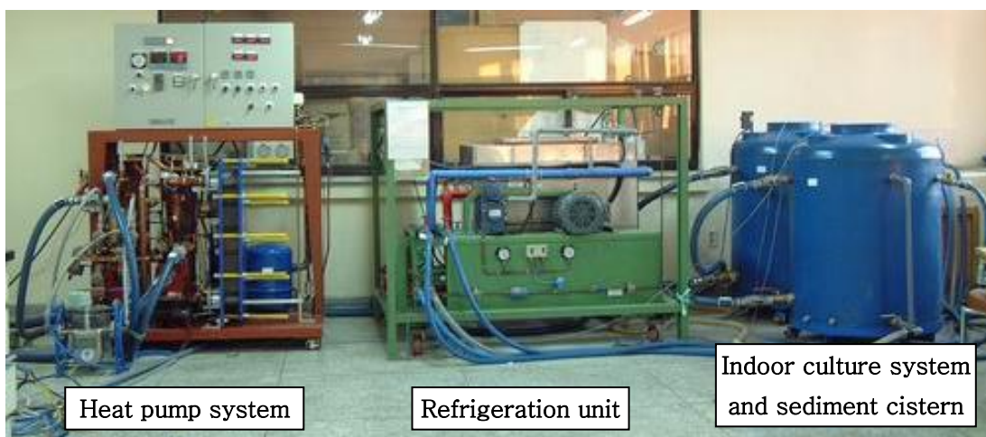
Photo 1. High efficient heat pump system with supply water volume 6 \text{ m}^3/\text{h} .
