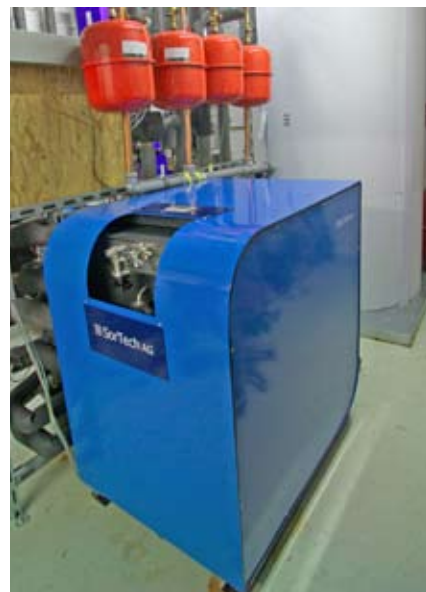
Adsorption chiller - cooling with solar heat in summer and heating as a thermally driven heat pump in winter
