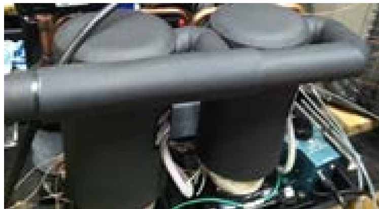
Figure 28: Insulated tandem compressors
