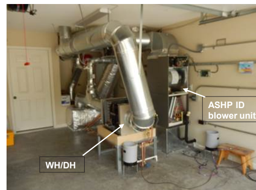
Figure 4. AS-IHP 2 field-test prototype in installation process.
