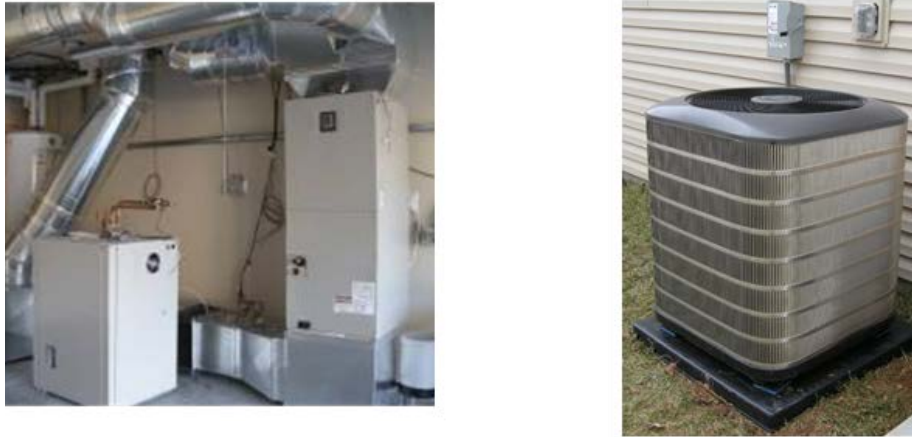
Figure 2. AS-IHP 1 field test prototype installation; left) indoor sections (hot water storage tank, compressor and water heating module, and indoor fan coil), right) outdoor section.
