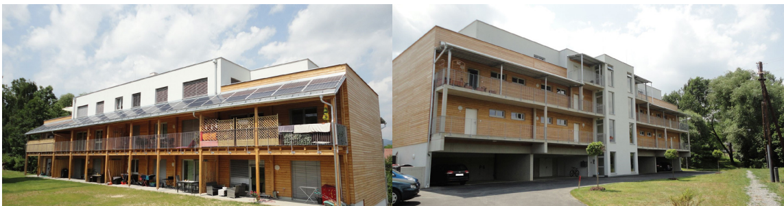
Figure 1. A multi-family building in Weiz, Austria which has been constructed in 2014/15. It consists of 10 apartments on three floors, a 957 m 2 heated floor area, and it conforms to the passive house standard (wood frame construction, floor heating system, controlled ventilation with heat recovery).
