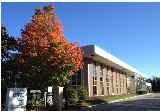
Figure 1. ASHRAE HQ, Atlanta, USA. A commercial building with an on-going monitoring program.
