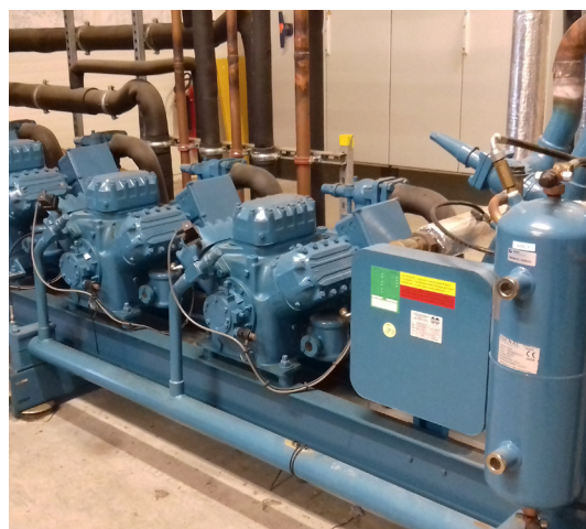
Figure 2. The refrigeration system of a supermarket is often used as a heat pump, also providing hot water and space heating for the sales area.
