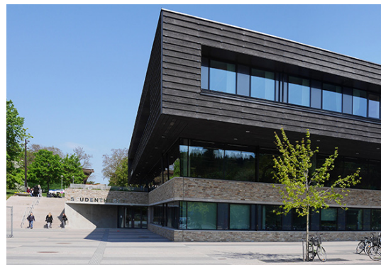
Figure 2. Studenthuset, Stockholm, Sweden. An institutional building with an on-going monitoring program.
