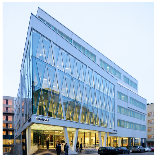
Figure 3. The Skanska HQ building in Stockholm, Sweden, uses the ground as a source for direct cooling, and for pre-heating of ventilation air.
