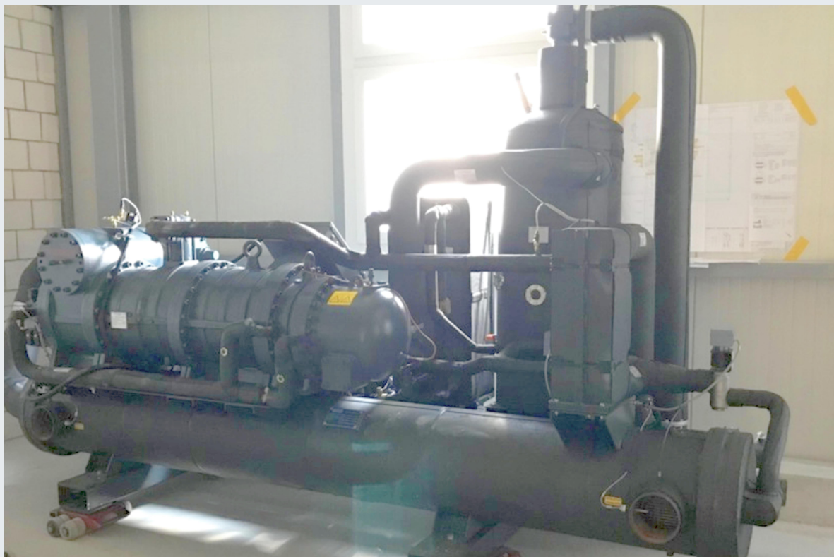
Fig. 2: High temperature heat pump installed at the technical room of the mountain cheese factory [4]. The mildly flammable refrigerant R1234ze(E) demands special measures for fire protection and escape routes.
