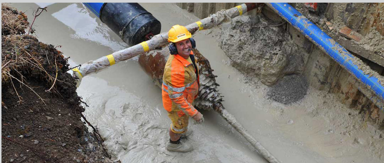
Fig 1: Picture of a trench, while laying the anergy network.
