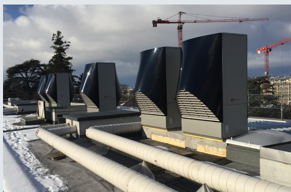
Figure 2: Two rooftop projects with air-to-water heat pumps realized in Geneva. Right: industrial heat pumps with over 80dB(a) at emission with surrounding noise-reduction walls (Source: SIG/ CSD Ingénieurs SA)
