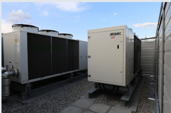
Figure 2: Two rooftop projects with air-to-water heat pumps realized in Geneva. Right: industrial heat pumps with over 80dB(a) at emission with surrounding noise-reduction walls (Source: SIG/ CSD Ingénieurs SA)
