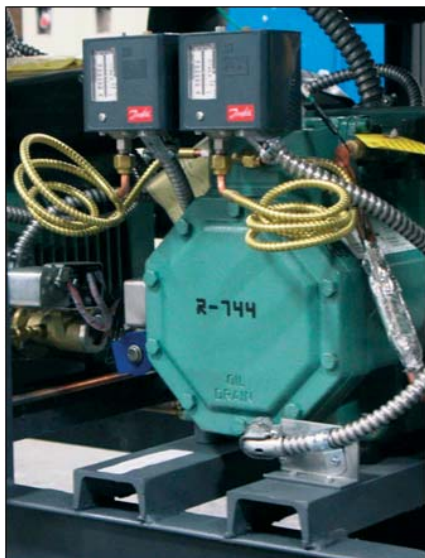
Figure 4. CO 2 Cascade Compressor
