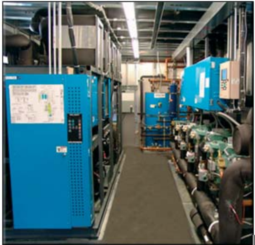
Figure 1. CO 2 Secondary Installation for a Wal-Mart Warehouse-Style Store
