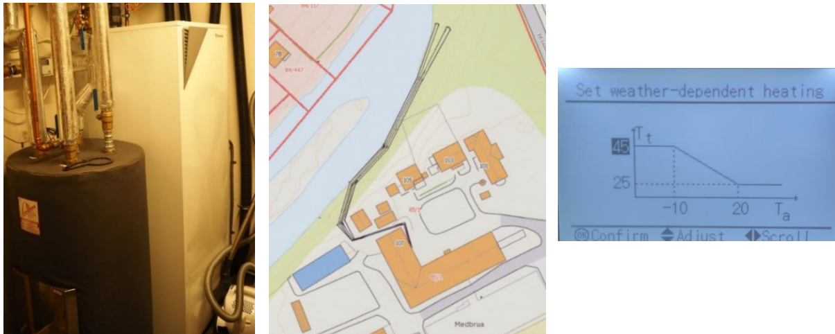
Figure 126: The technical room showing the accumulation tank, the heat pump unit and some of the connected pipes (left, Rønneseth, 2017). Ambient temp. compensation curve for the heat pump (picture of display) (middle, Rønneseth 2017). Location of the pipes for the horizontal ground collector system (right, Thyholt, 2014).
