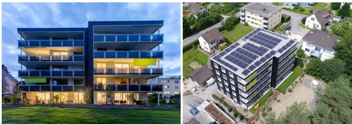
Figure 61: Back-view of the building Sonnenpark Plus with façade integrated PV in the balcony (left) and air-view with roof integrated PV-system
