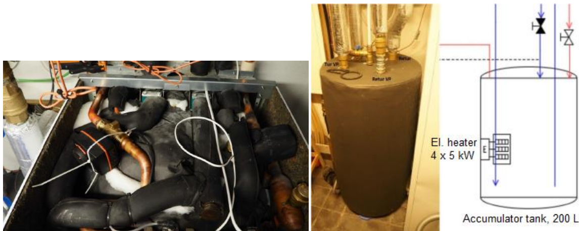
Figure 130: Top of the heat pump, where the shuttle valve is mounted with a strip (left) and accumulator tank (middle) and segment from the principle sketch (right) (Rønneseth, 2017)
