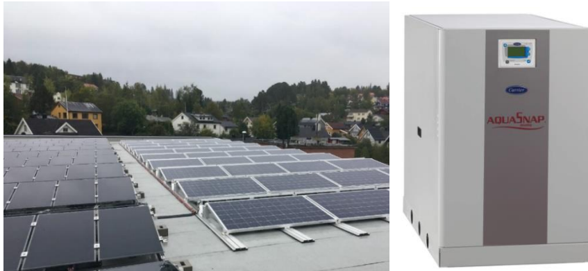
Figure 133: PV on the roof-top of KIWI Dalgård, with thin film PV on the left and crystalline PV on the right (left, Aaberg, 2018) and Heat pump unit, Carrier Aqua Snap 61WG (right, AHI Carrier, 2018).
