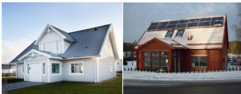
Figure 15: Twin houses, i.e. two almost identical nZEB buildings with same building envelope, but different heat pump system installed
