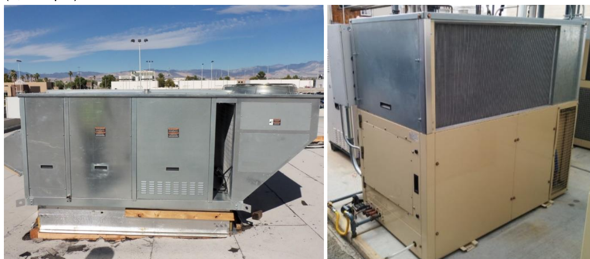
Figure 57: Commercial gas engine AS-IHP installed on the roof at the field demonstration site and final version of the prototype residential gas engine AS-IHP.
