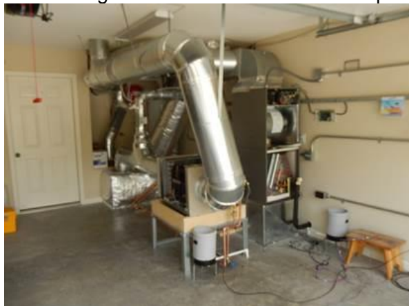
Figure 52: Field-test prototype during installation. ASHP indoor air handler and WH/DH prototype shown with rain gauges for condensate collection to monitor DH and latent cooling loads (left) and schematic of coaxial tank water fitting
