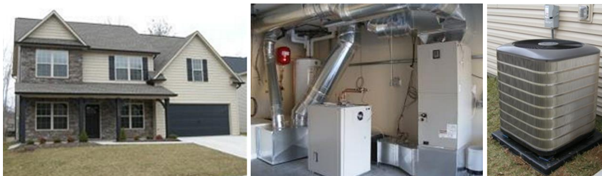
Figure 48: Field test site in Yarnell Station neighborhood, Knoxville, Tennessee (left), Prototype installation: indoor sections (HW storage tank, compressor and water heating module, and indoor fan coil) (middle) outdoor fan coil section (right)
