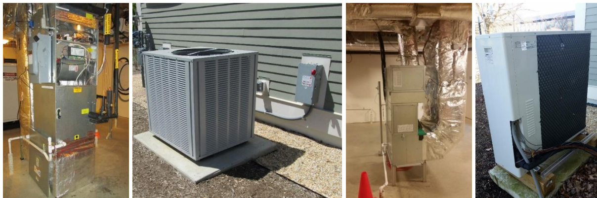
Figure 64: CDHP system indoor and outdoor units at NZERTF: indoor air handler (left) and outdoor unit (mid left) and SDHV system indoor and outdoor units at NZERTF: indoor air handler (mid right) and outdoor unit (right).
