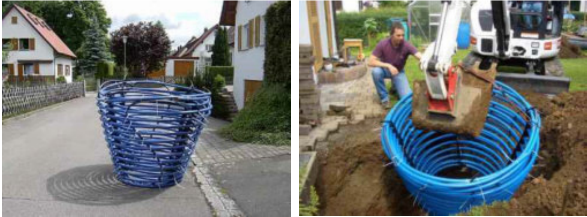
Fig. 3: Ground basket heat exchanger coil
