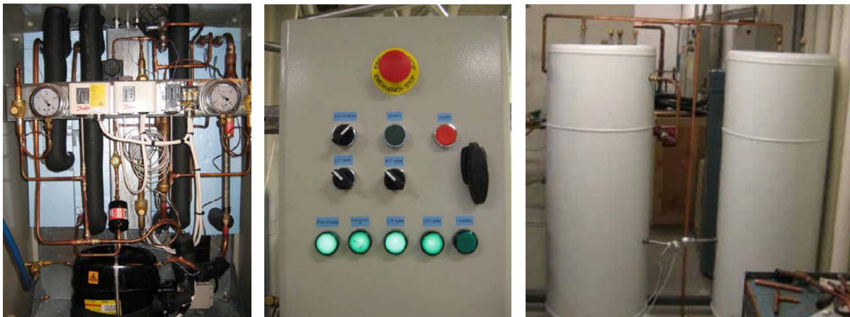
Fig. 54: Prototype heat pump, cabinet for the electrical equipment and storage tanks
