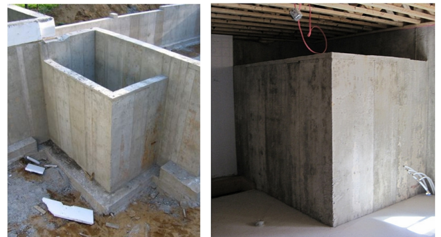
Integrated concrete thermal energy storage for space heating and DHW preheating
