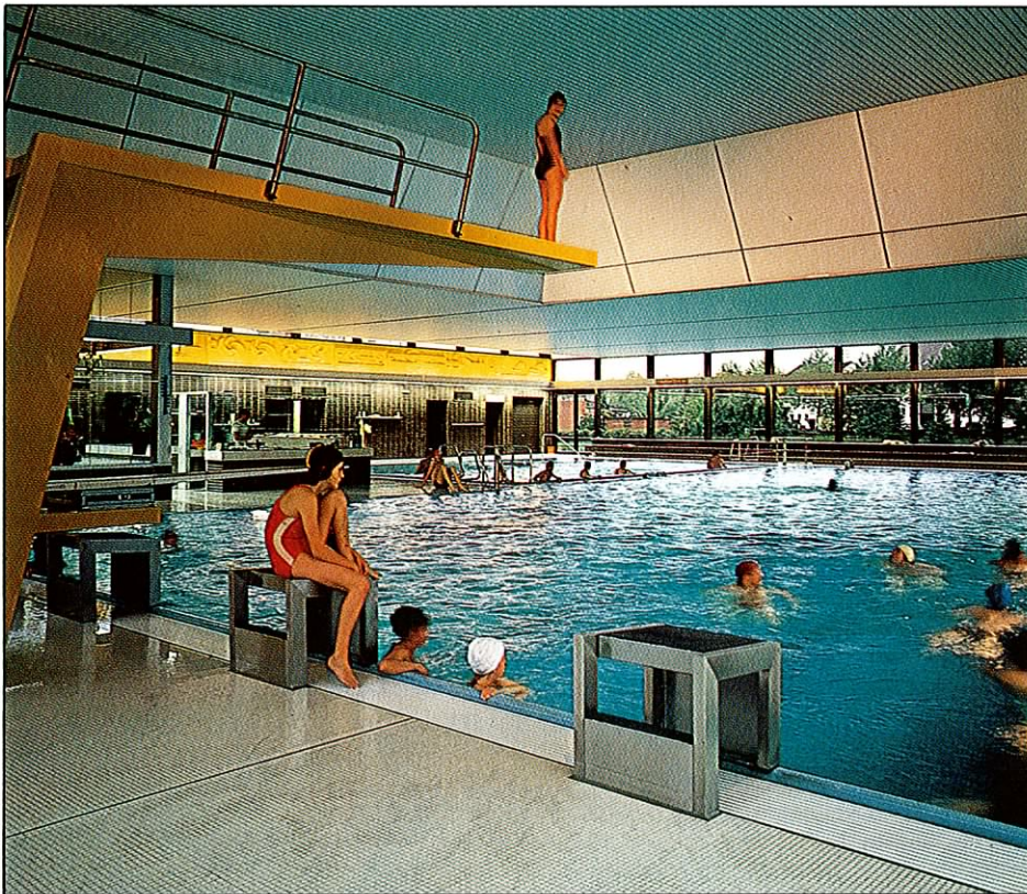
Indoor Swimming Pool Heated by Electrically Driven Heat Pump at Forchheim near Karlsruhe. Photograph by Bauer/Badenwerk.
